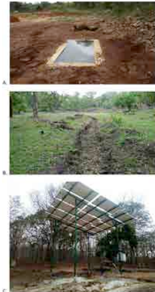
Image 3. Measures suggested from the findings of this study and their implementation: A—Construction of smaller artificial water tanks and fill them with water tankers | B—Removing obstructing bigger shrubs surrounding major waterholes before every rainy season so that more and more water gets accumulated in waterholes | C—Installation of solar powered pumping bore wells near major waterholes at feasible locations in the forest.
