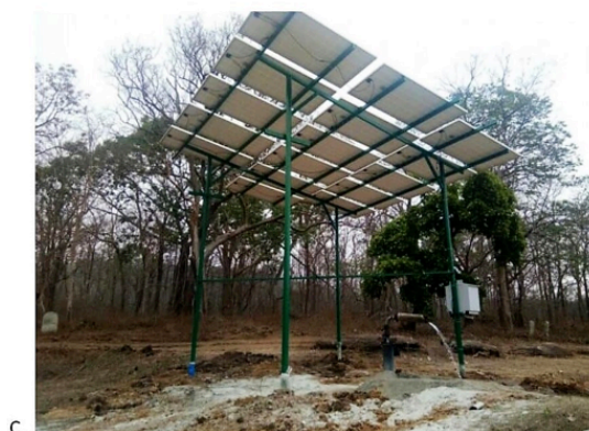
Image 3. Measures suggested from the findings of this study and their implementation: A—Construction of smaller artificial water tanks and fill them with water tankers | B—Removing obstructing bigger shrubs surrounding major waterholes before every rainy season so that more and more water gets accumulated in waterholes | C—Installation of solar powered pumping bore wells near major waterholes at feasible locations in the forest.
